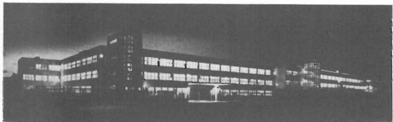
Night view of the L. M. Ericsson Works from the post-office
